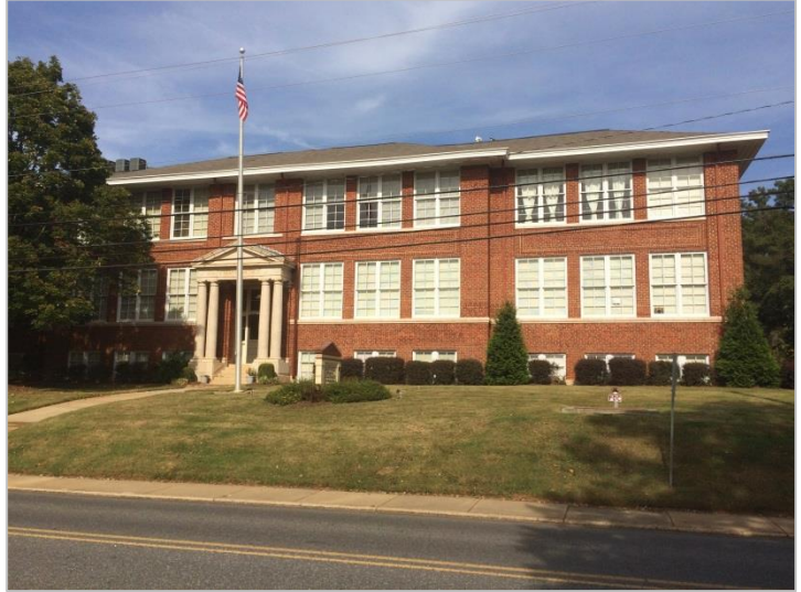
Mayworth School (AECOM, 2018)
