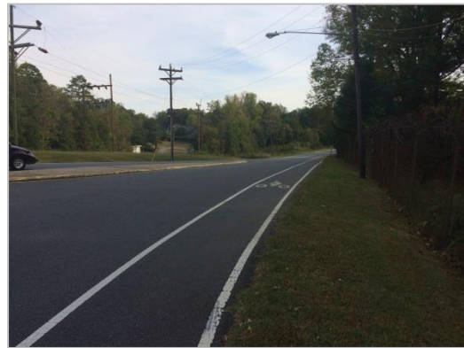
Eastwood Drive near Eagle Road in Cramerton (AECOM, 2018)
