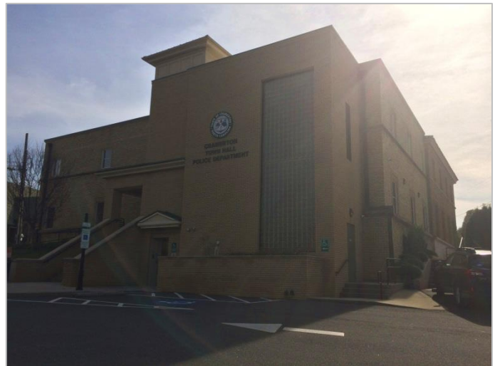
Cramerton Town Hall (AECOM, 2018)
